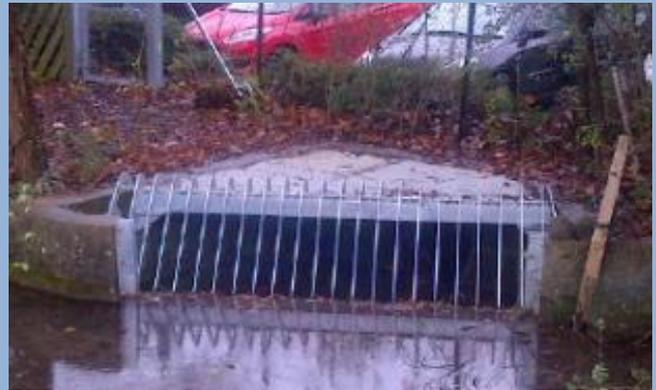
Above: The new trash pins at Studio Culvert (left) and the new trash screen on the Tesco Culvert (right)
